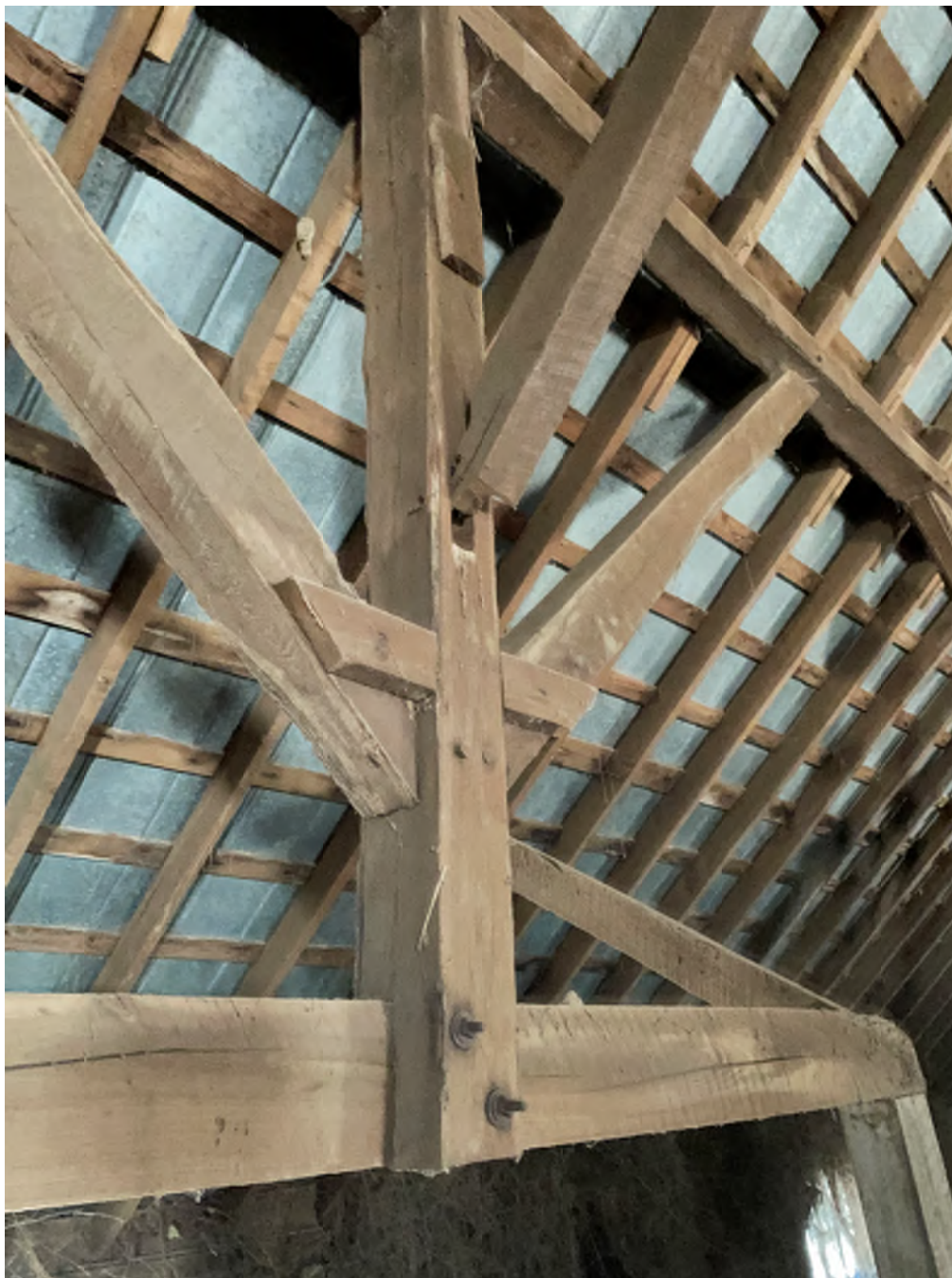
Transferred post to be stabilized.
