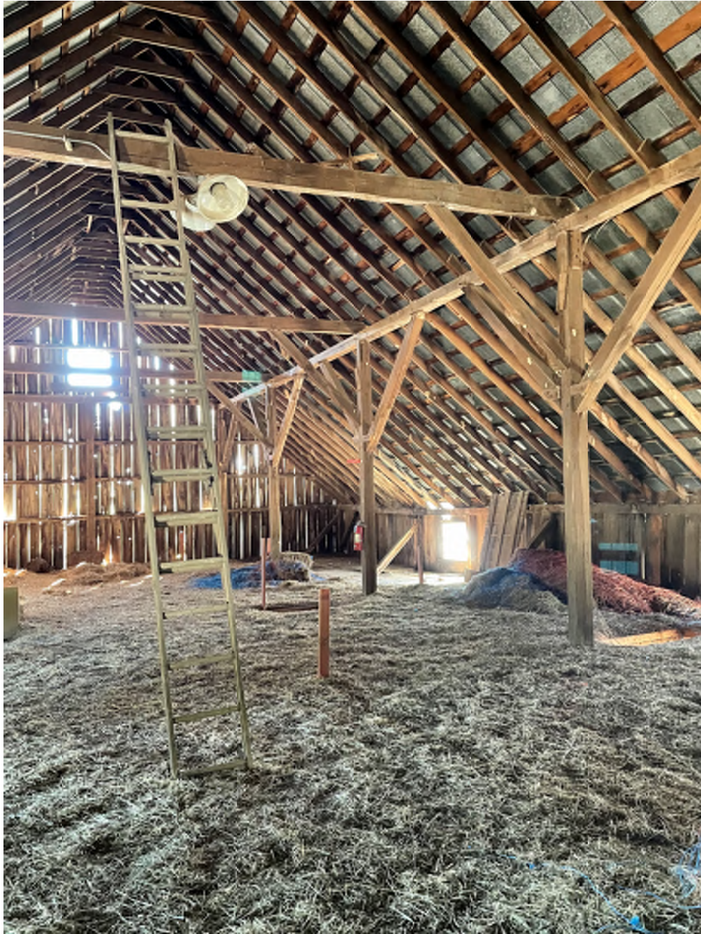
View of loft framing. Small posts on the floor indicate openings.
