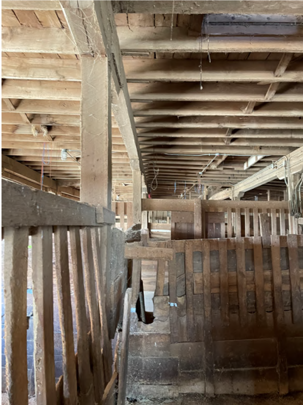
Note limited internal bracing.
